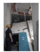
Damage from Hydrogen Build Up
